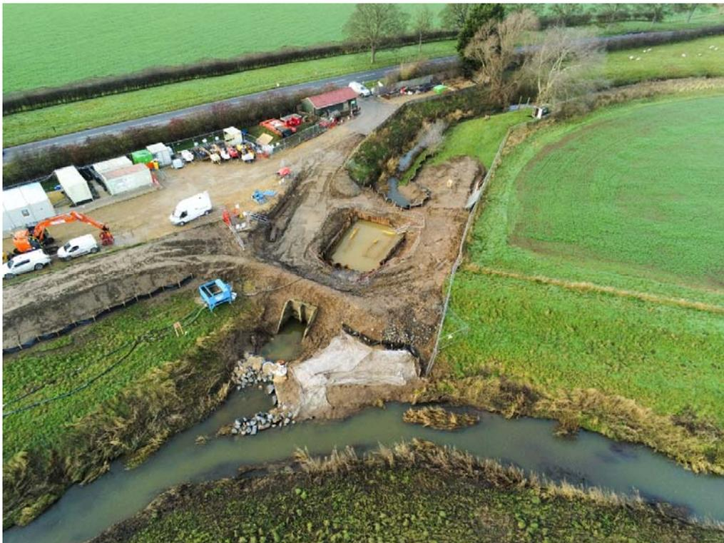
The upstream flow control structure remains in place while the new structure is built slightly upstream. This is allowing us to deliver the Flood Warning Service as normal. Once the new structure is built and gauging equipment installed we will be able to remove the existing structure. The River Leven flow is being managed as normal with the flow control penstocks being closed when we are expecting high flows in the Leven.
