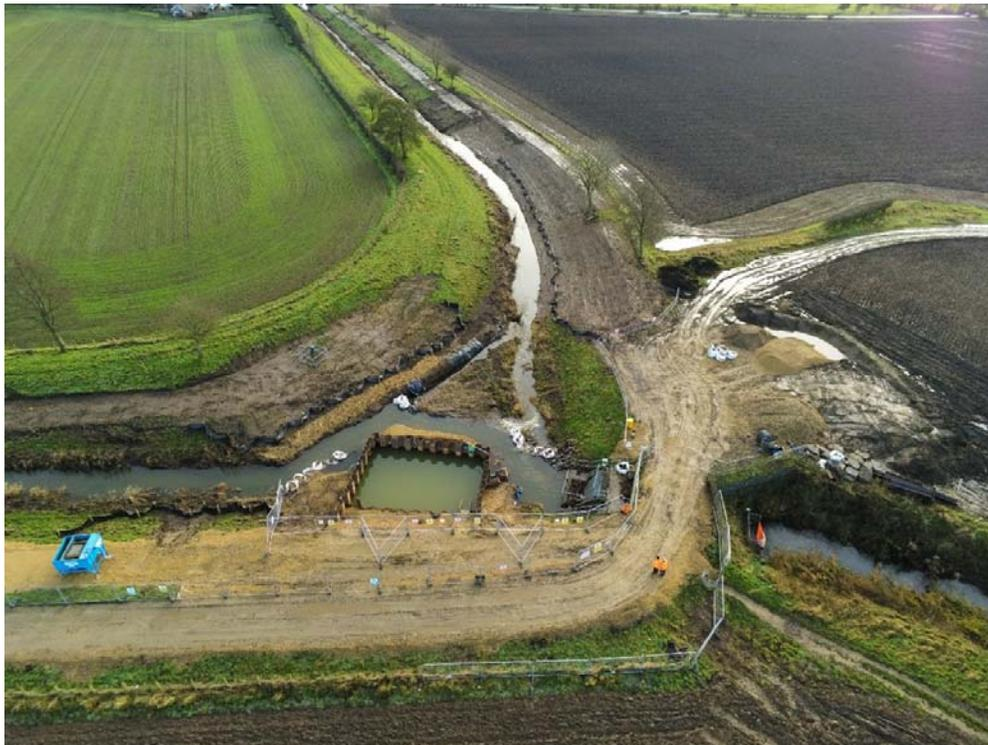
The flood diversion channel is being re-profiled to ensure it has the capacity to contain flows and make maintenance easier and safer in the future. This requires some tree management and will result in some trees being removed.
